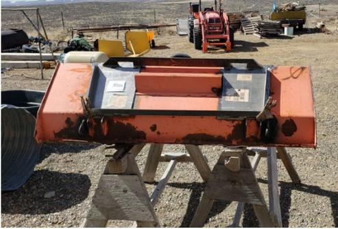
The weld-on plate has been stabilized with clamps and tack welded. Note how the angle iron support brace has been maintained inside the weld-on plate. It won't be in the way of the quick attach.
