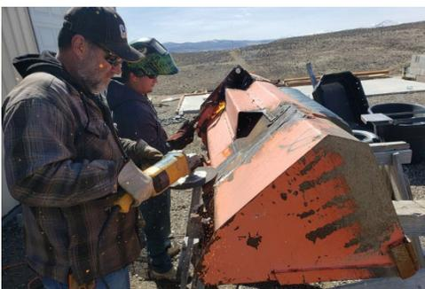
As you can see in our pictures, one old pin-on bracket has been removed and the remaining material is being removed with a grinder. You can also remove the pins with a cutting torch.
